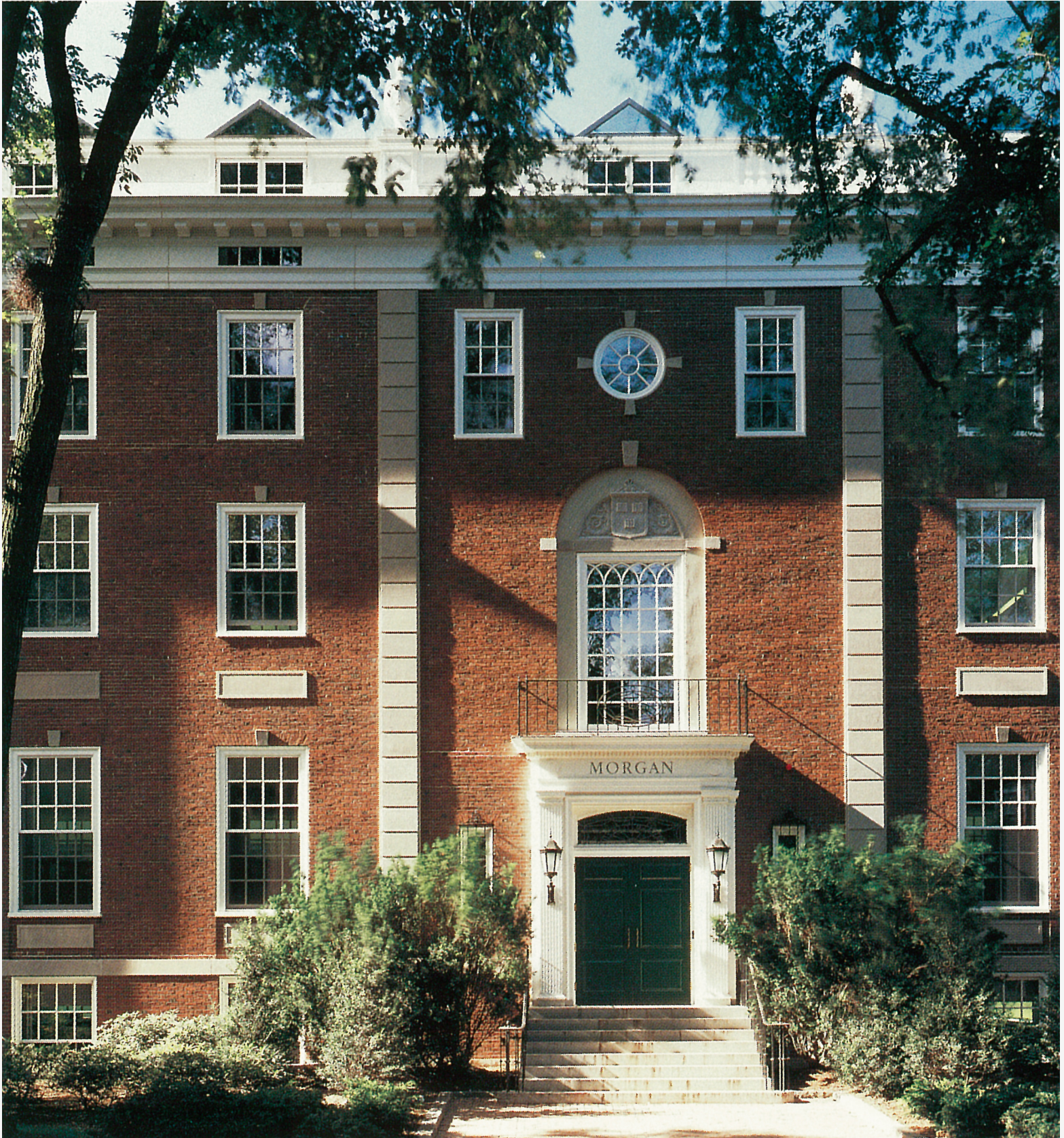
Morgan Hall, Harvard Business School 1 Elevation view
