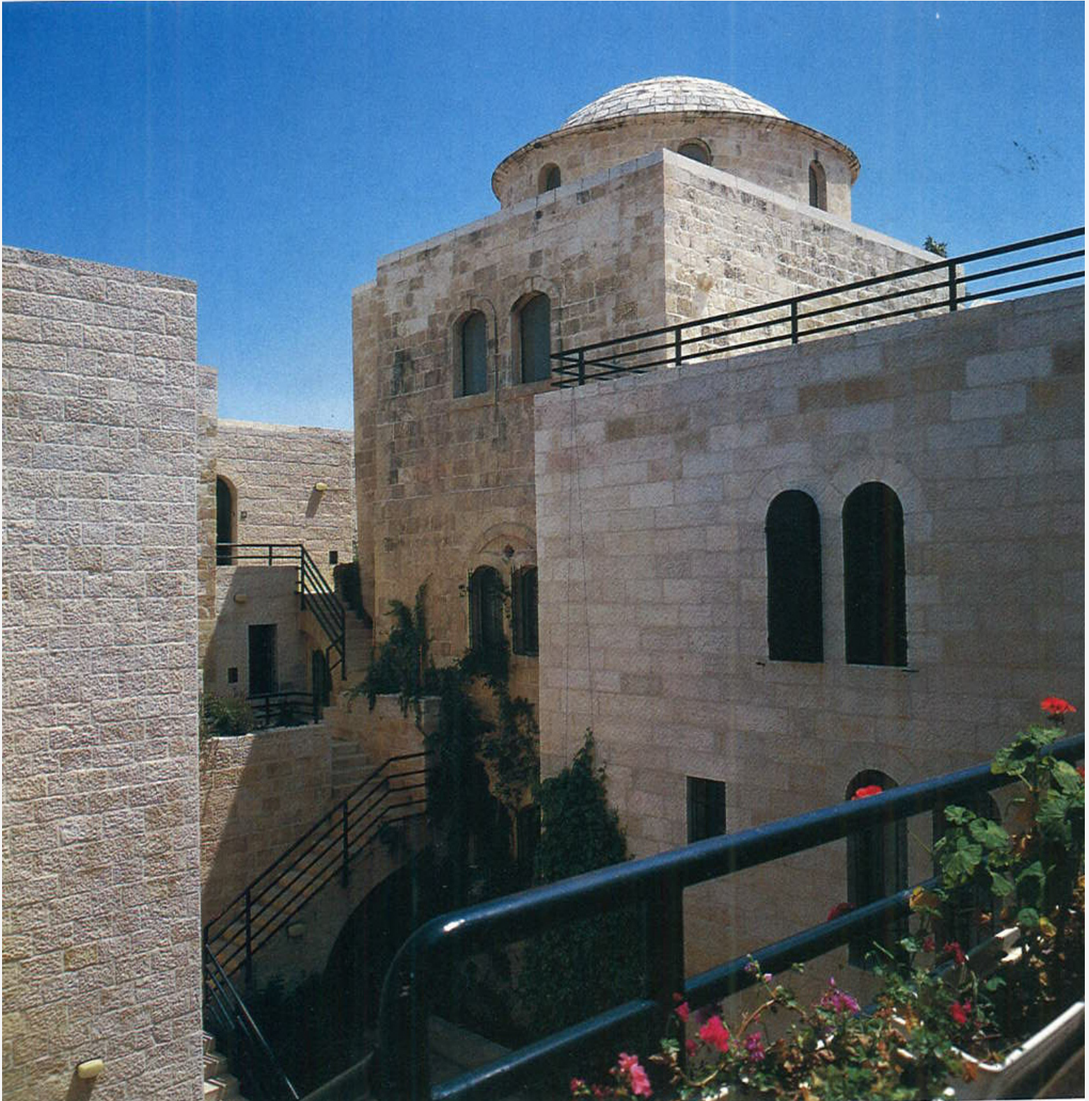
Hosh District 1 Wall detail
